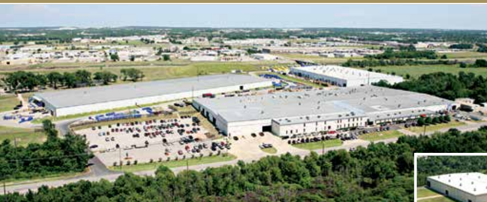
Ameristar's world headquarters, manufacturing & coil processing facilities in Tulsa, Oklahoma, USA.
